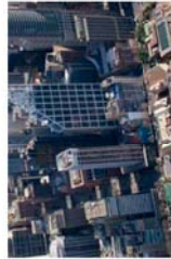
Figure 3. Aerial, copyright airview online
